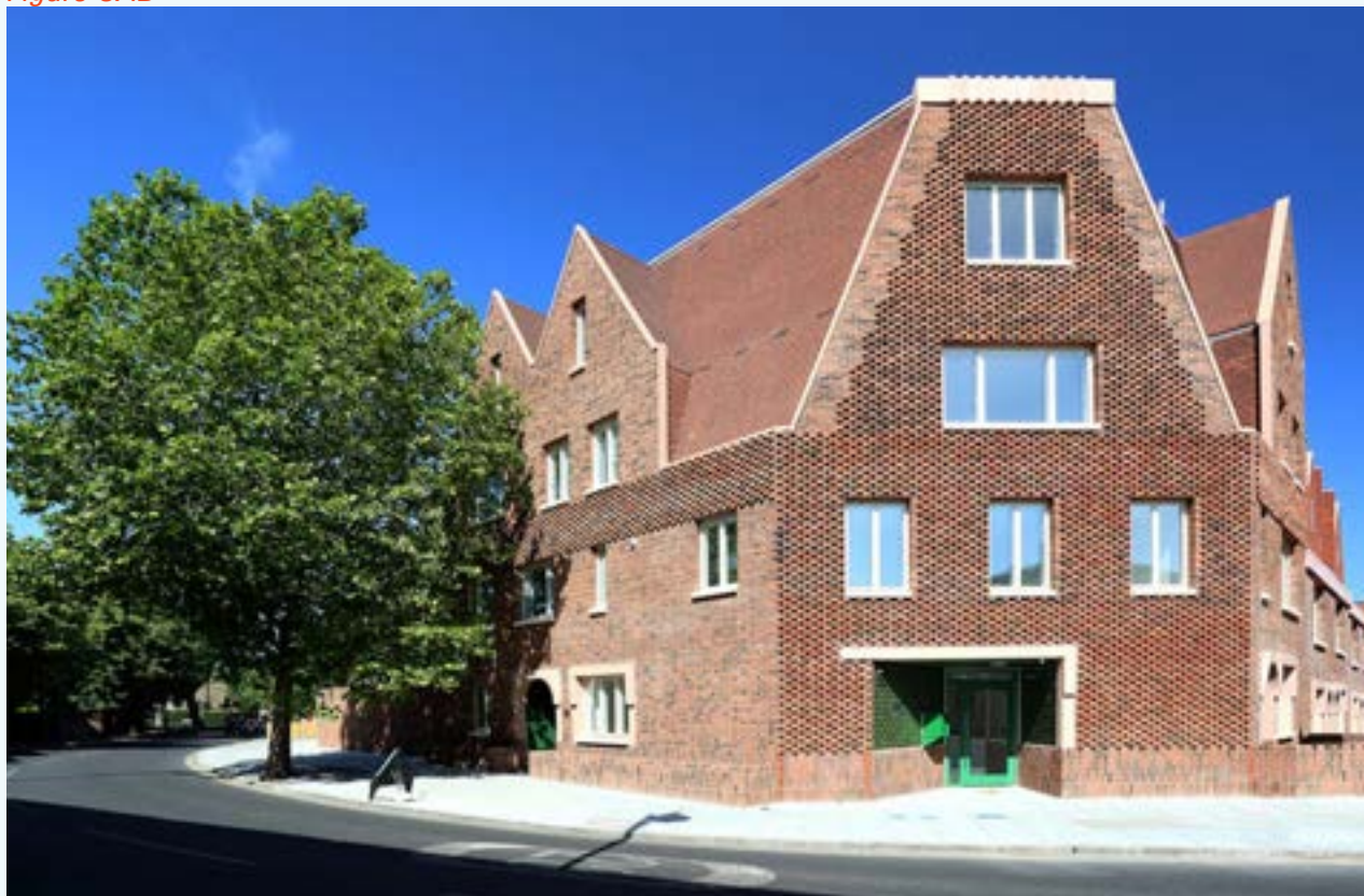
Nunhead Green in Southwark by AOC and David Miller Architects show how roof forms can be used to articulate the top of a four-storey apartment building.
